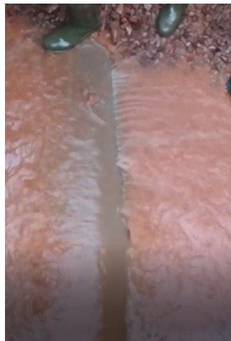
Excavation at the leak location
